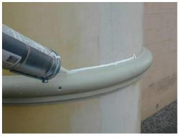
16) Apply a bead of good paintable exterior chalk at the top and bottom joint where the neck ring joins the column. Smooth bead for proper appearance.
