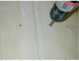
3) Reinstall pan head screws on the column half just assembled with adhesive.
