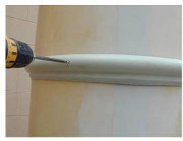
9) Using the 1-3/4" self-drilling screws, install the first neck ring half to the column, lining up the line to the bottom of the neck ring.
