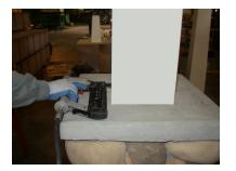
10) Nail column to post ONLY ON THE BOTTOM . Do not attach at center or top (to allow for expansion).
