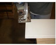
2) PVC expands and contracts with temperature changes. Trim shaft pieces to 1/2" shorter than opening height (from step 1) to allow for product expansion.
